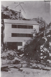
17. Sandbekk: subsidiary building south-west of dressing plant; aerial ropeway in background.
