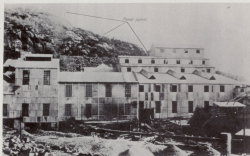
15. Sandbekk: grinding and concentration plant.
