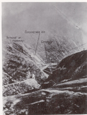
18. Jödingfjorden: view of concentrate storage and shipping installations, looking southward from above the west side of the head of the fjord.
