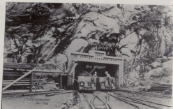
12. Sandbakki: entrance of main haulage drive (exact site not located).
