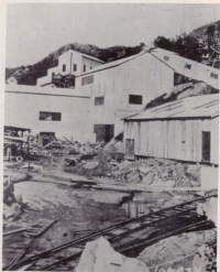
13. Sandbakk: Intermediate crushing installation; grinding and concentration plant in left background.
