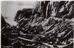
7. Jösingfjorden: view down the fjord from road north-east of Nedre Helleren, showing on the right, Sogndal road and tunnels.
