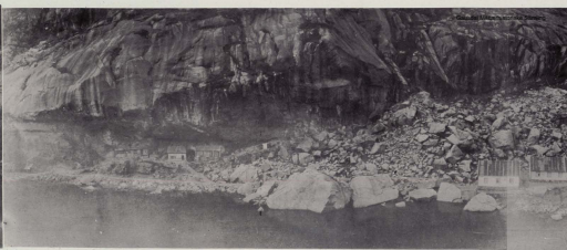
3. Jösingfjorden: the head of the fjord, showing disused zinc factory, Nedre Helleren power station and workers' dwellings. Old herring oil factory at Holmen on extreme left. The rails seen in left foreground were used in constructing the coastal road to Holmen.
