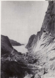
6. Jösingfjorden (1937): view down the fjord from road north-east of Nedre Helleren; taken when Sogndal road and tunnel (extreme right) were under construction.
